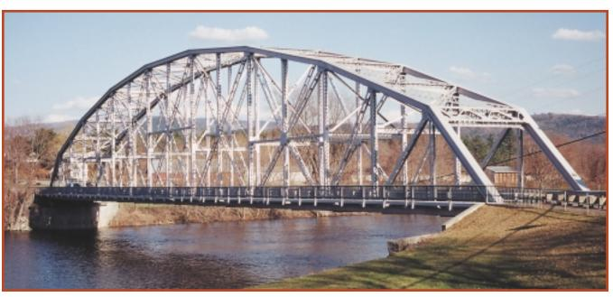
One of the most dramatic bridges constructed after the 1927 flood was the 352-foot Pennsylvania truss span over the Connecticut River from Piermont to Bradford, Vermont, completed in 1929.
