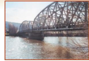
*The two-span, 459-foot Parker truss bridge between Lyme and Thetford, Vermont was completed in 1937.*
