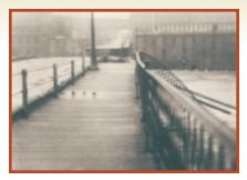
This photo of the McGregor Bridge in Manchester was taken as the span began to break up during the floods of 1936. As debris from this bridge was swept downstream, the Amoskeag Steam Pipe Bridge was also destroyed.
